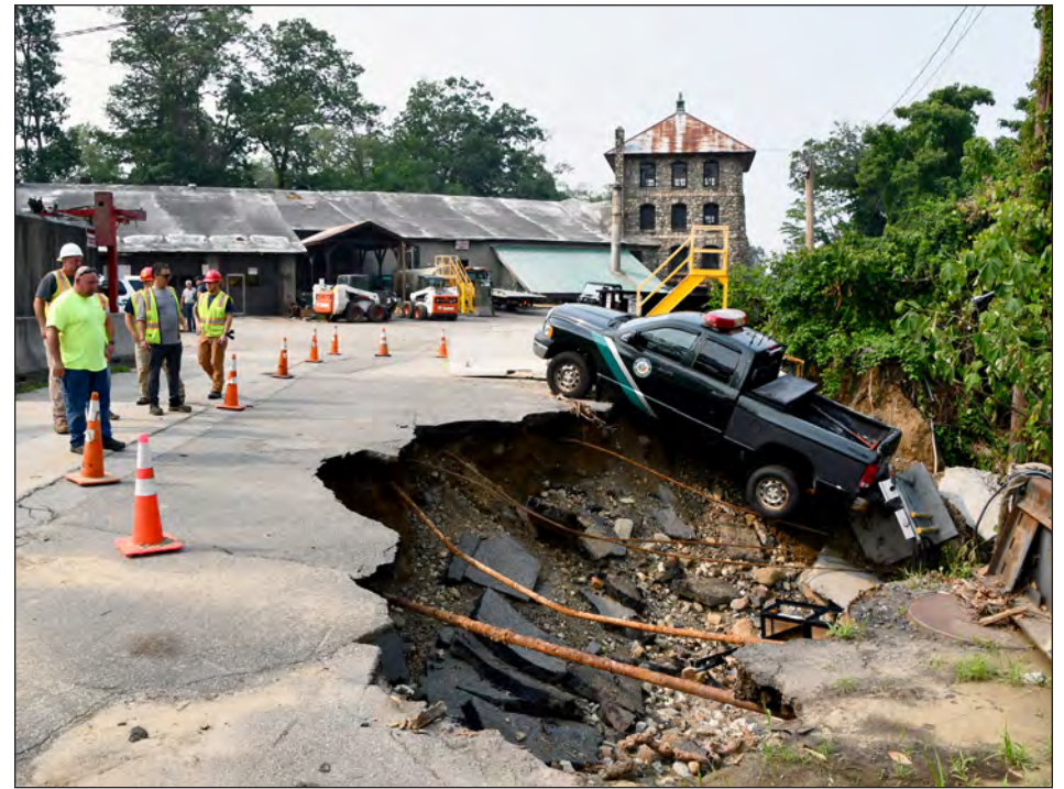
Cristian Gonzalez, front left, observes flooding damage to the road, vehicles and equipment at Bear Mountain State Park.
