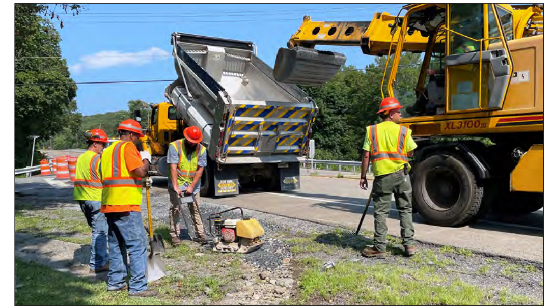
Town of Cornwall Unit member Michael Cwikla, left, and Unit Vice President Brenden Doyle work to redirect future water flow down the side of Old West Point Road in Cornwall. The flooding that hit the area on July 9 created the need for numerous road repairs and excavation.
